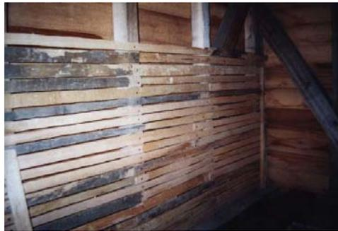
Below is a section of a lathe and plaster wall face on. You can see the pink plaster, which is pushed onto and into the yellow lathes, which in turn are fixed at narrow spacing to the upright timber studs.
